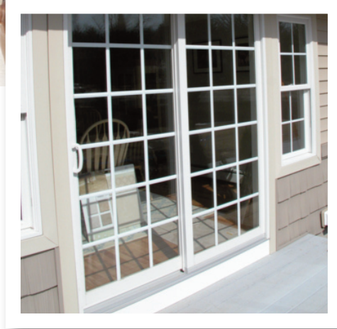
Optional grids are placed inside the insulated glass units, making cleaning a breeze.
